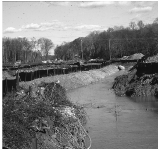
Figure 1. Silt fence placed along the banks of an existing stream.
