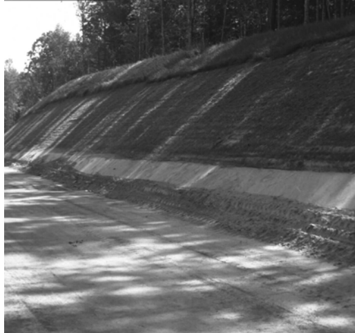
Figure 2. Slope grooved for seeding.
